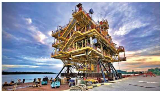
Well Head Topside Platform ready for Sail-away
