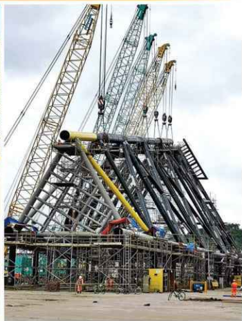
Heavy Lifting of Jacket Structure
