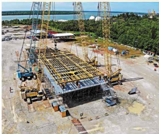
Heavy Lifting of Cellar Deck Structure
