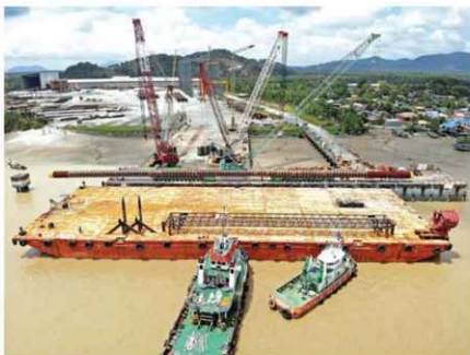
Load-out of Piles and Conductors
