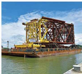
Sail-away of Jacket Structure
