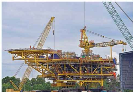
Load-out of Well Head Platform with Helideck
