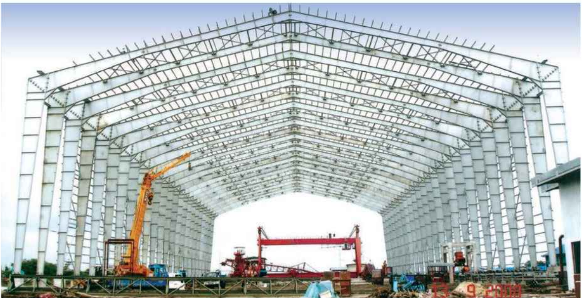
Mukah Coal-Fired Power Station, Mukah (2008)
