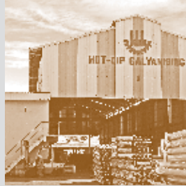
Hot-Dip Galvanising plant setup
