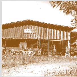
Small welding workshop
