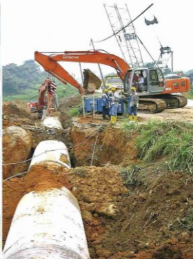
1600mmND Steel Pipeline from Jalan Batu Kitang to Jalan Datuk Stephen Yong / Jalan Batu Kawa Junction, Kuching (2003)
