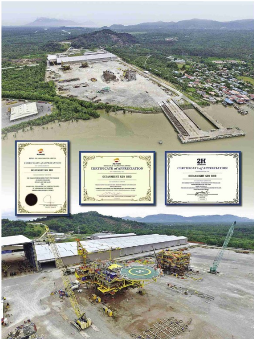
Strategic fabrication yard with deep water jetties and loadout capacity of up to 30,000 metric tones
