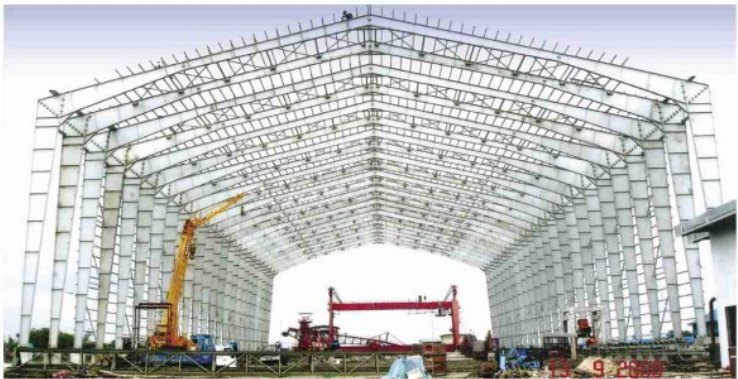
Mukah Coal-Fired Power Station, Mukah [2008]
