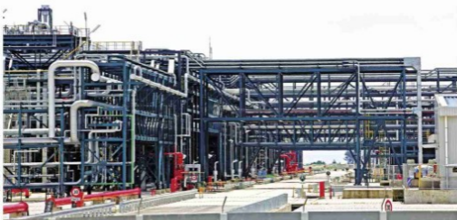
Polycrystalline Silicon Manufacturing Plant for Tokuyama Malaysia at Samalaju Industrial Park, Bintulu (2011)
